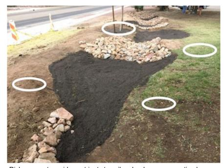
Rich compost provides nutrients to soil and reduces evaporation loss from well-constructed water harvesting depressions. Rock spillways direct overflow water from one depression to the next, slowing water and reducing soil erosion. Potential tree-planting sites (circles) next to depressions allow trees to benefit from soil nutrients and harvested water.
