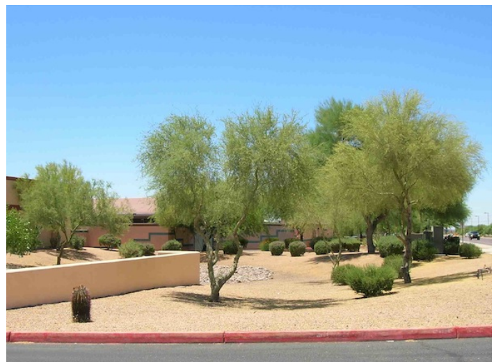
A gently sloped landscaped stormwater management basin at a commercial site receives runoff from building roofs and the parking lot, supporting native edible trees.
