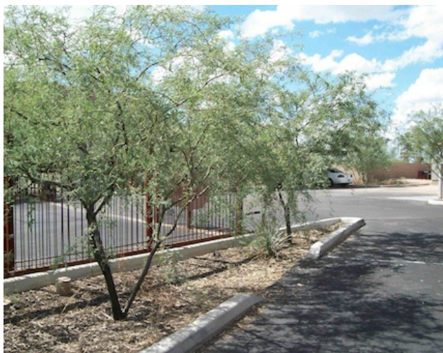
A curb cut leads runoff water from a parking lot to an adjacent depression planted with native trees.
