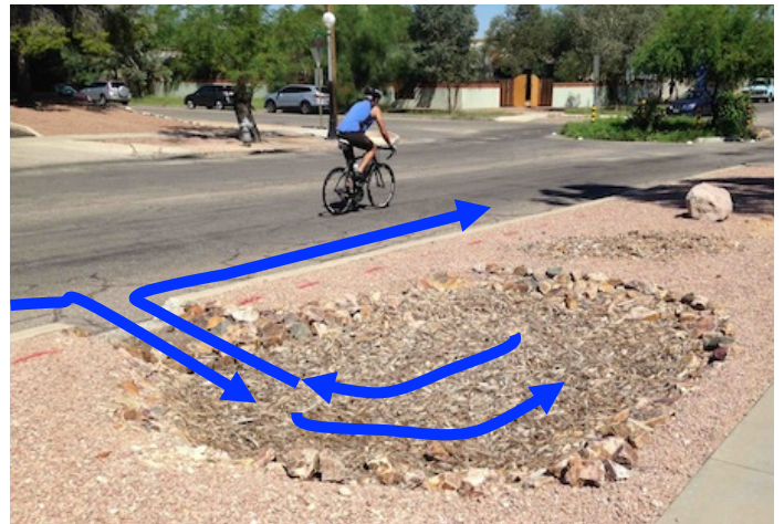
A newly constructed water harvesting basin will receive street runoff through a curb cut. Water flowing down the street curb will enter the basin through a narrow channel. When the basin is full, surplus water will exit back out the same channel to rejoin flow on the street.
