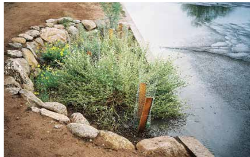
Street runoff flows down along the curb and gently through a curb cut to an adjacent planting basin, supporting growth of native edible shrubs.
