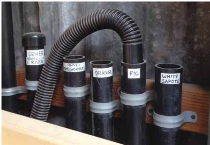
The owner of an outdoor washing machine discharges graywater to a different pipe with each wash. Each pipe drains to a different edible tree. The soaps used are made for graywater systems.
