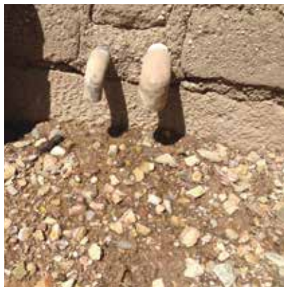
Air conditioner condensate water runs out of a pipe onto the soil next to a house (left). One cup of water can be harvested from this pipe every five minutes (right) by attaching a hose and running it to a nearby edible tree.
