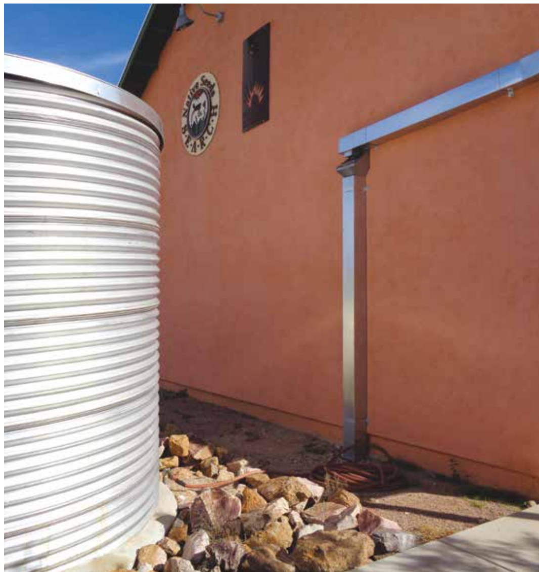
Large rainwater tank is filled from the adjacent gutter and downspout, harvesting water from a large roof. Water is piped down the wall in a water-tight downspout, then through an underground pipe and up into the tank. Tank is tapped with a hose bib. Water is delivered to adjacent landscape via gravity flow using a garden hose. Tank is positioned away from the building foundation in case the tank should leak.
