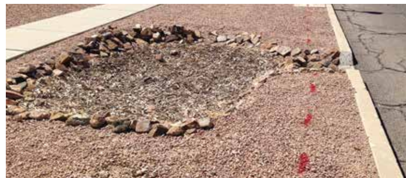
An underground utility line is marked here in red. Always determine the location and depth of buried lines before you dig. Use extreme caution when digging near buried utilities.
