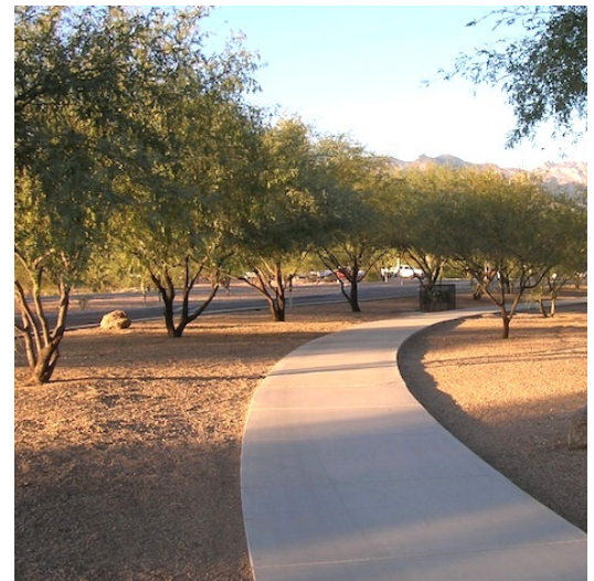
In a public park, well-spaced native edible trees are accessed by a raised sidewalk that provides rainwater runoff to the adjacent trees.
