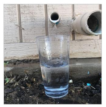
Water dripping from an ice machine condensate outlet fills a water glass.
