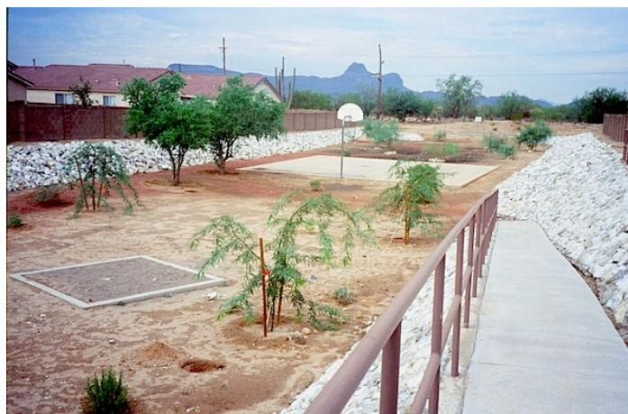
A multipurpose stormwater basin located in a residential subdivision manages large volumes of stormwater, supports low water-use edible trees and serves as a recreational areas residents can use during dry periods.
